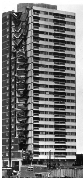
Figure: Damage caused by explosion
